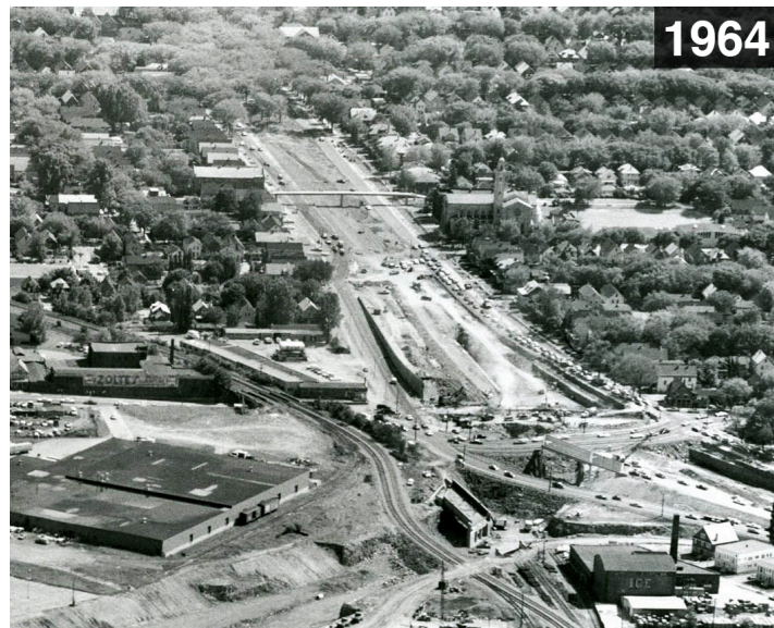
Figure 12 shows the construction of the Kensington Expressway. 84
