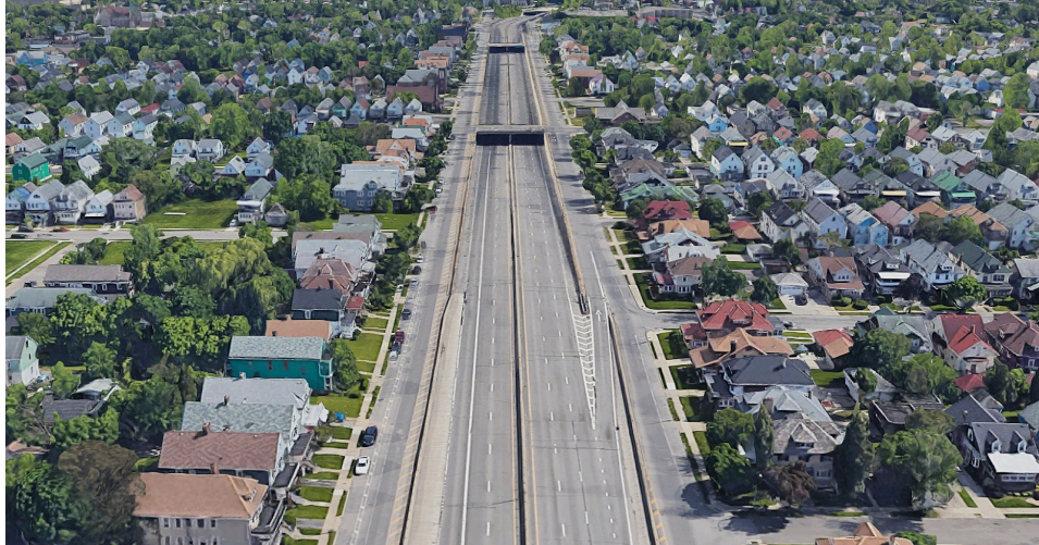
Figure 13 shows the current state of the Kensington Expressway. 85
